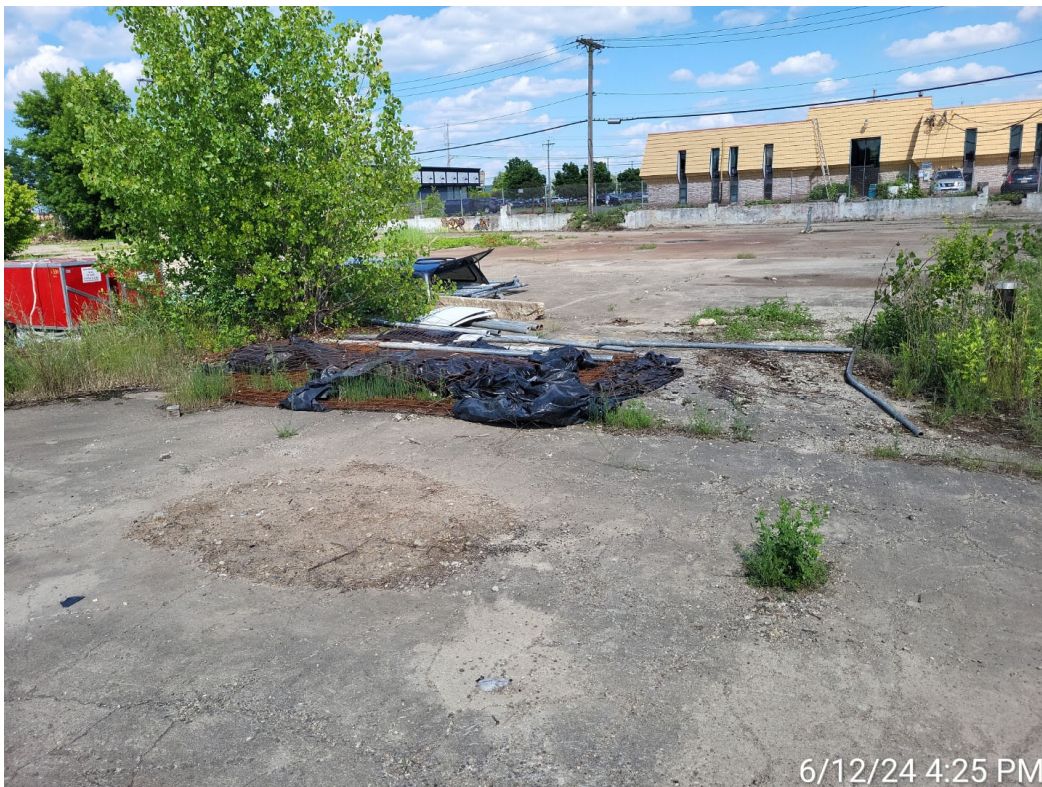
Debris is still onsite
