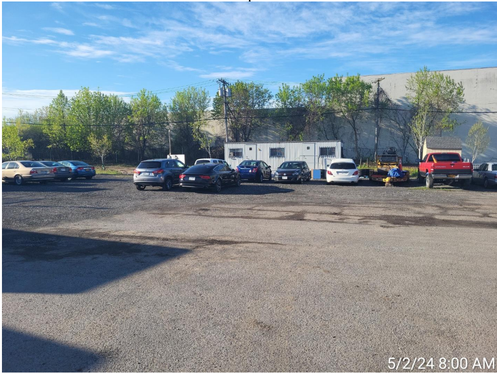
Job trailer on site. Electrical panel to the west of the trailer
